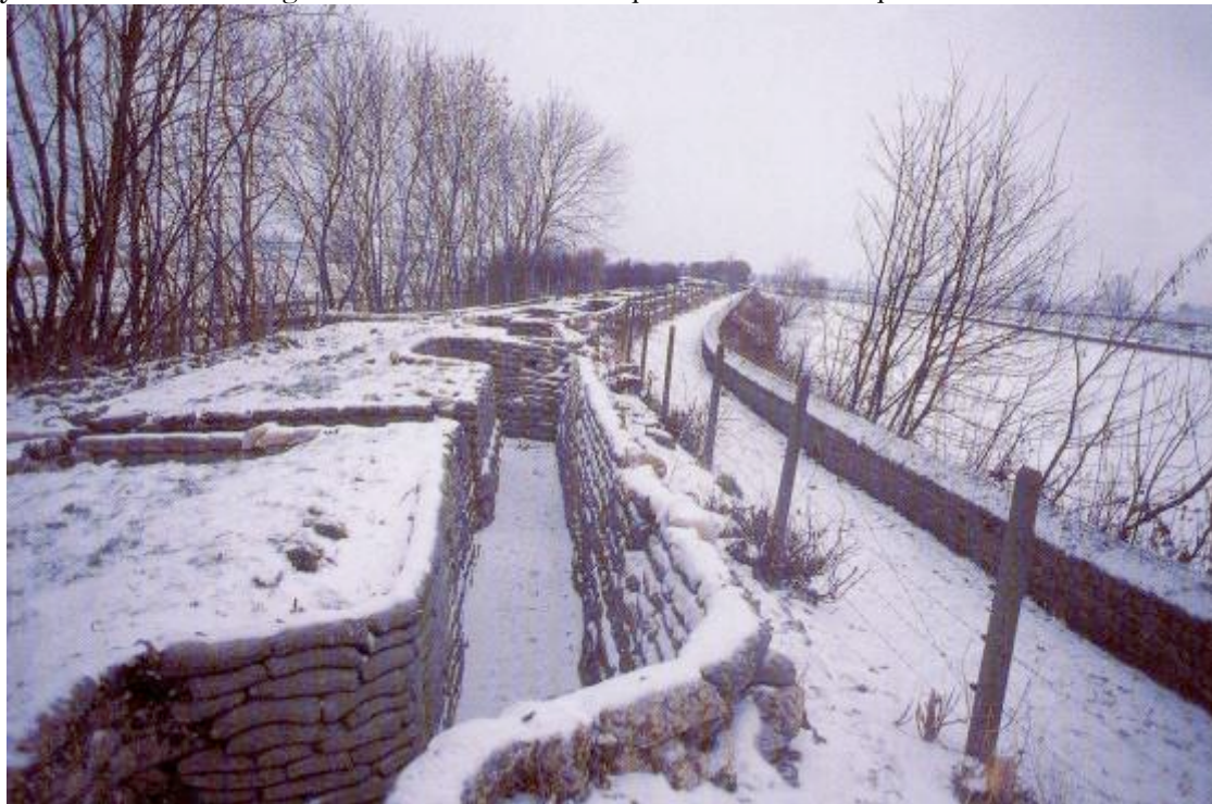
Trench by the canal
